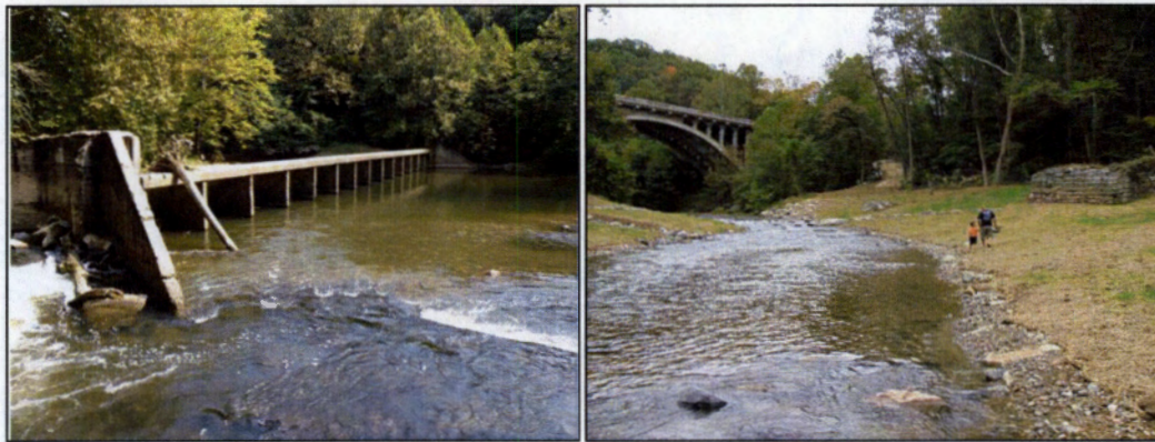
Figure 4: Union Dam site before and after dam removal
